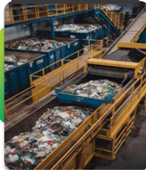
Waste plant Treatment
